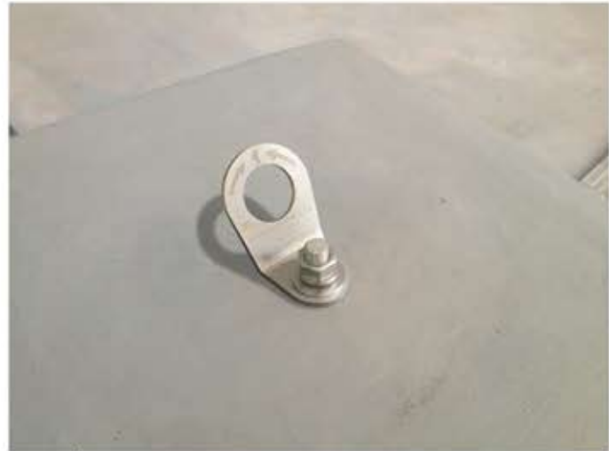
AKROPOINT INSTALLED ON CONCRETE
