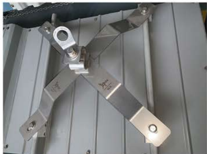
AKROPOINT INSTALLED ON METALLIC ROOF
